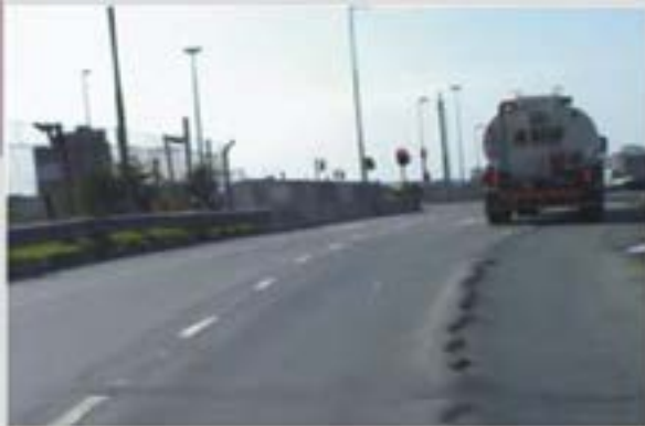
Figure 1(a). Severe rutting caused by heavy vehicles
